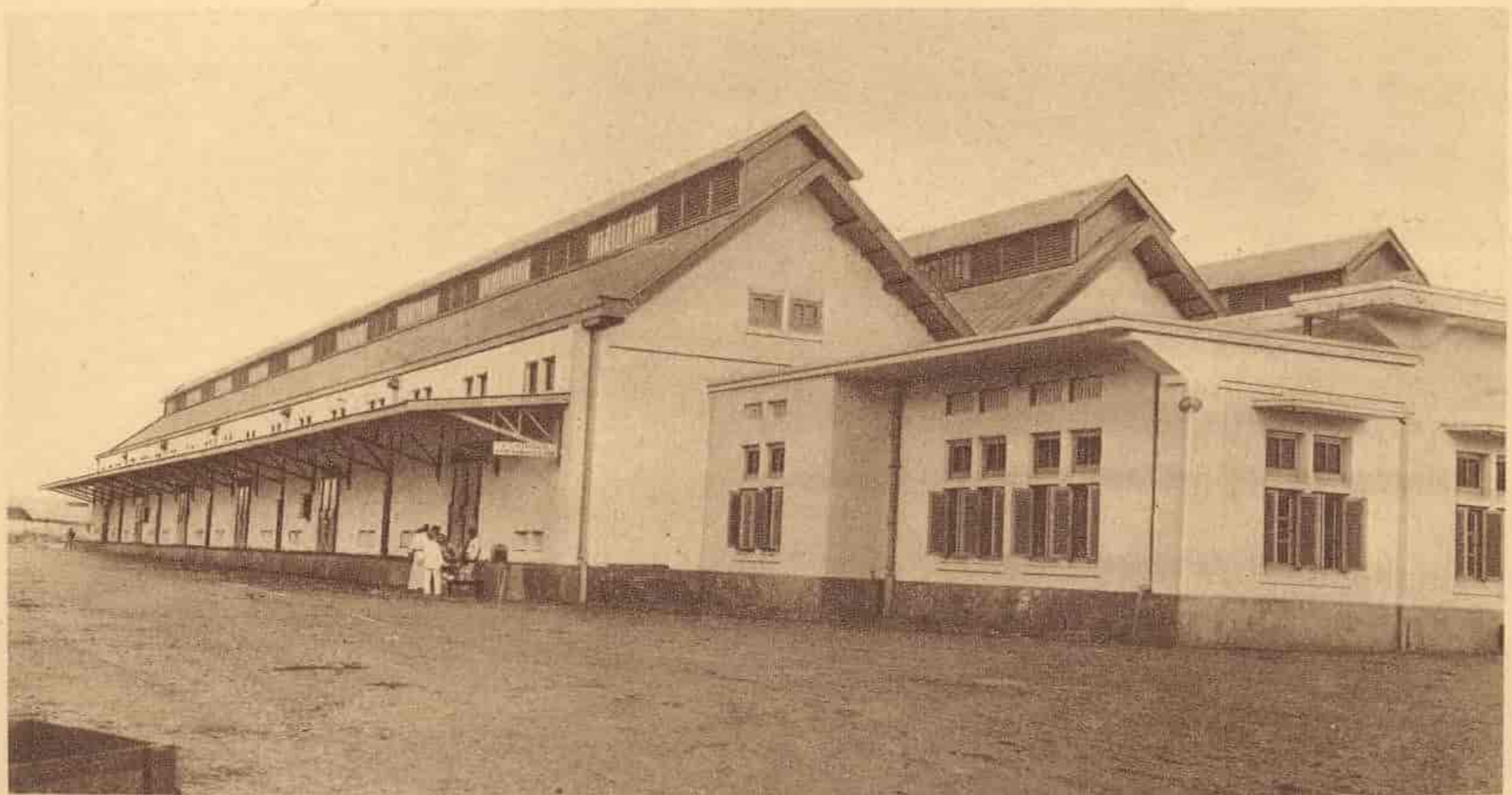
Station barang-barang jang baroe di Tjirojom (Bandoeng), selagi dibikin.
