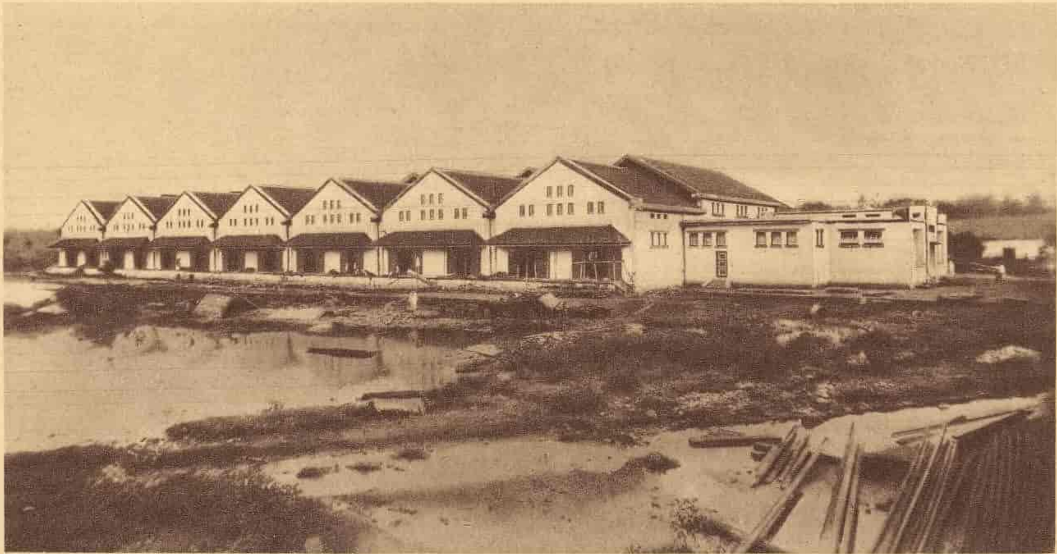
Station barang-barang jang baroe di Heemradenplein (Betawi) selagi dibikin.
