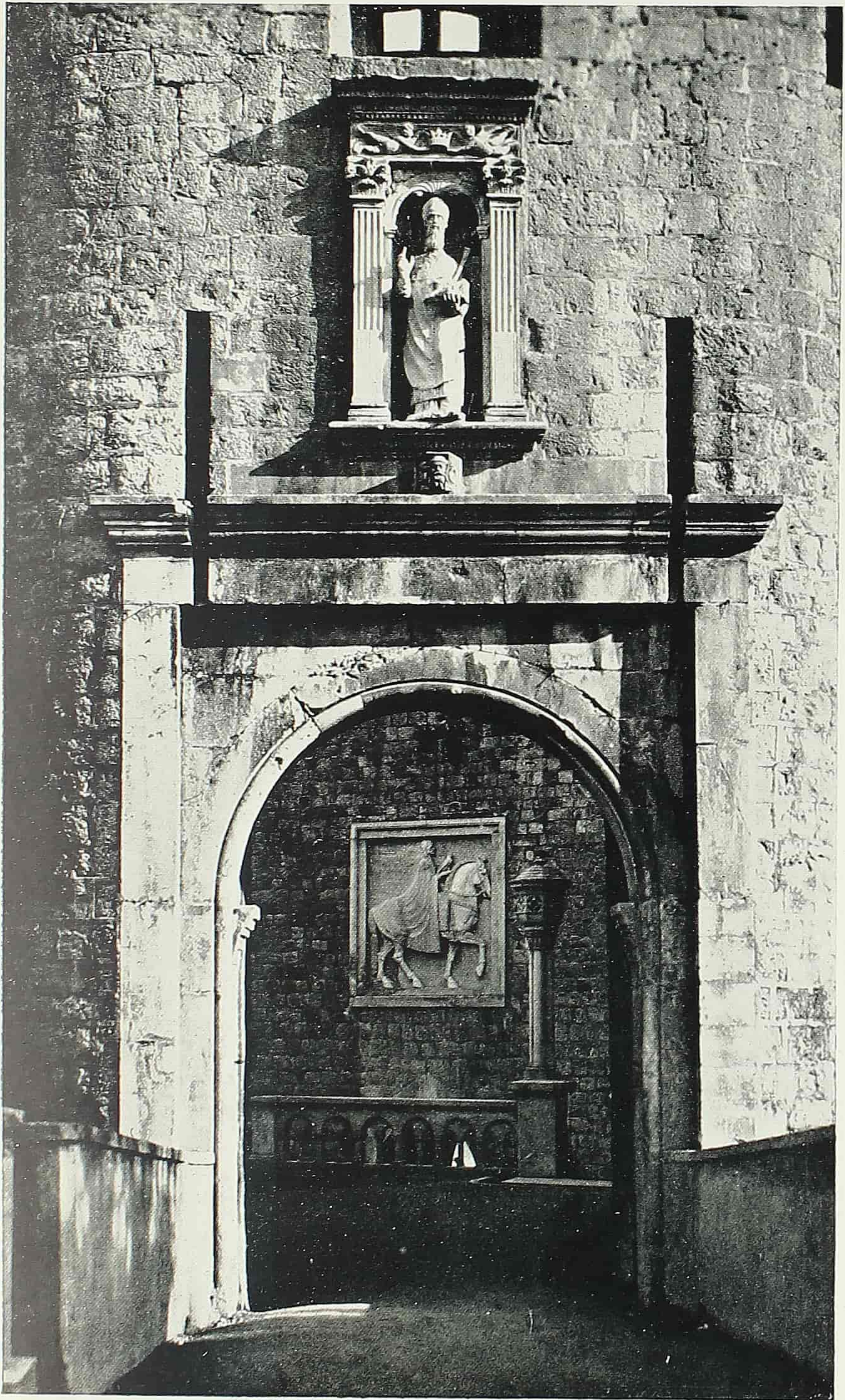
Dubrovnik, City gate of Pile
