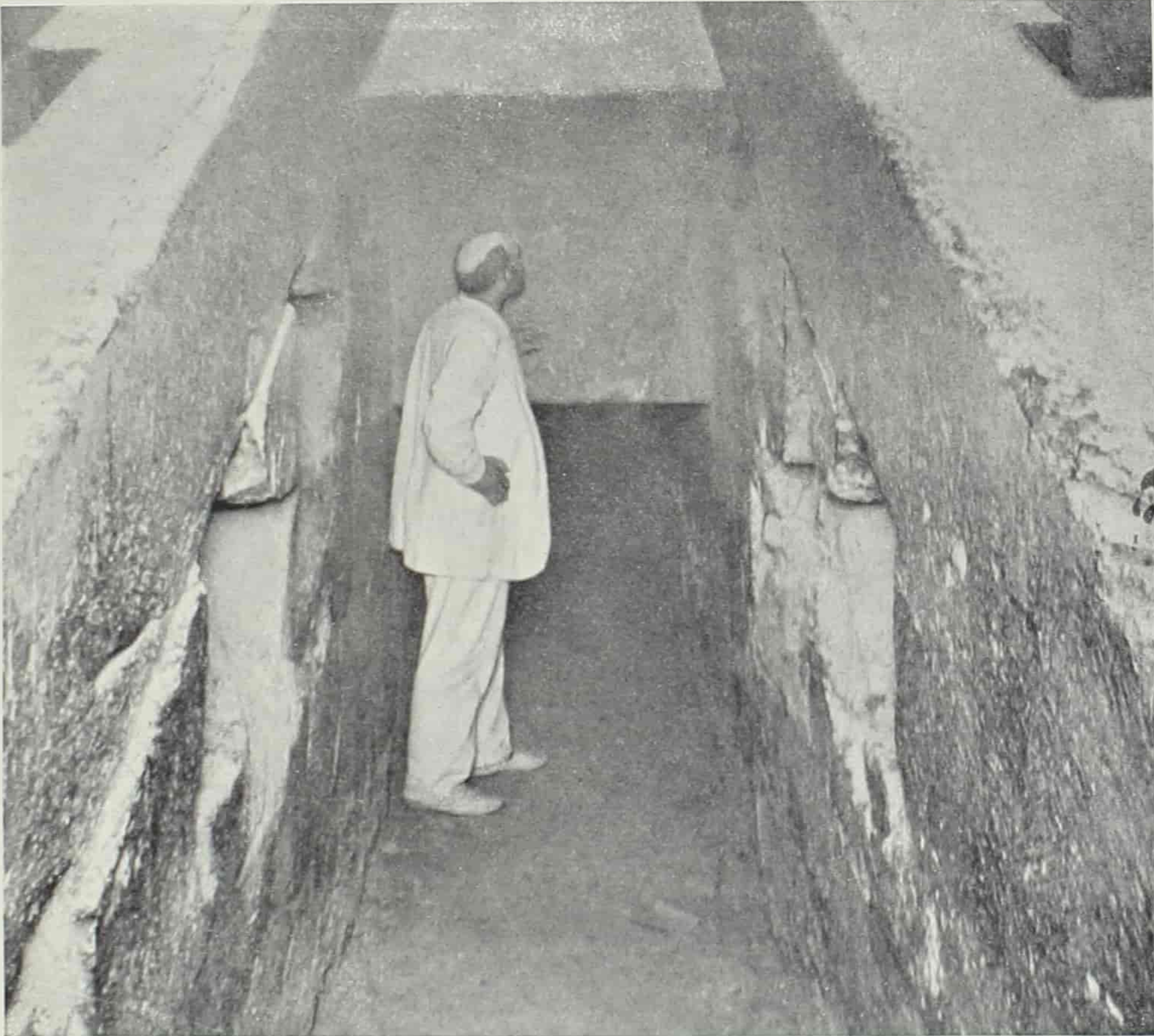
The entrance of the Horizontal Passage to the Queen's Chamber; showing the sheer-cut-off of the Grand Gallery floor.
