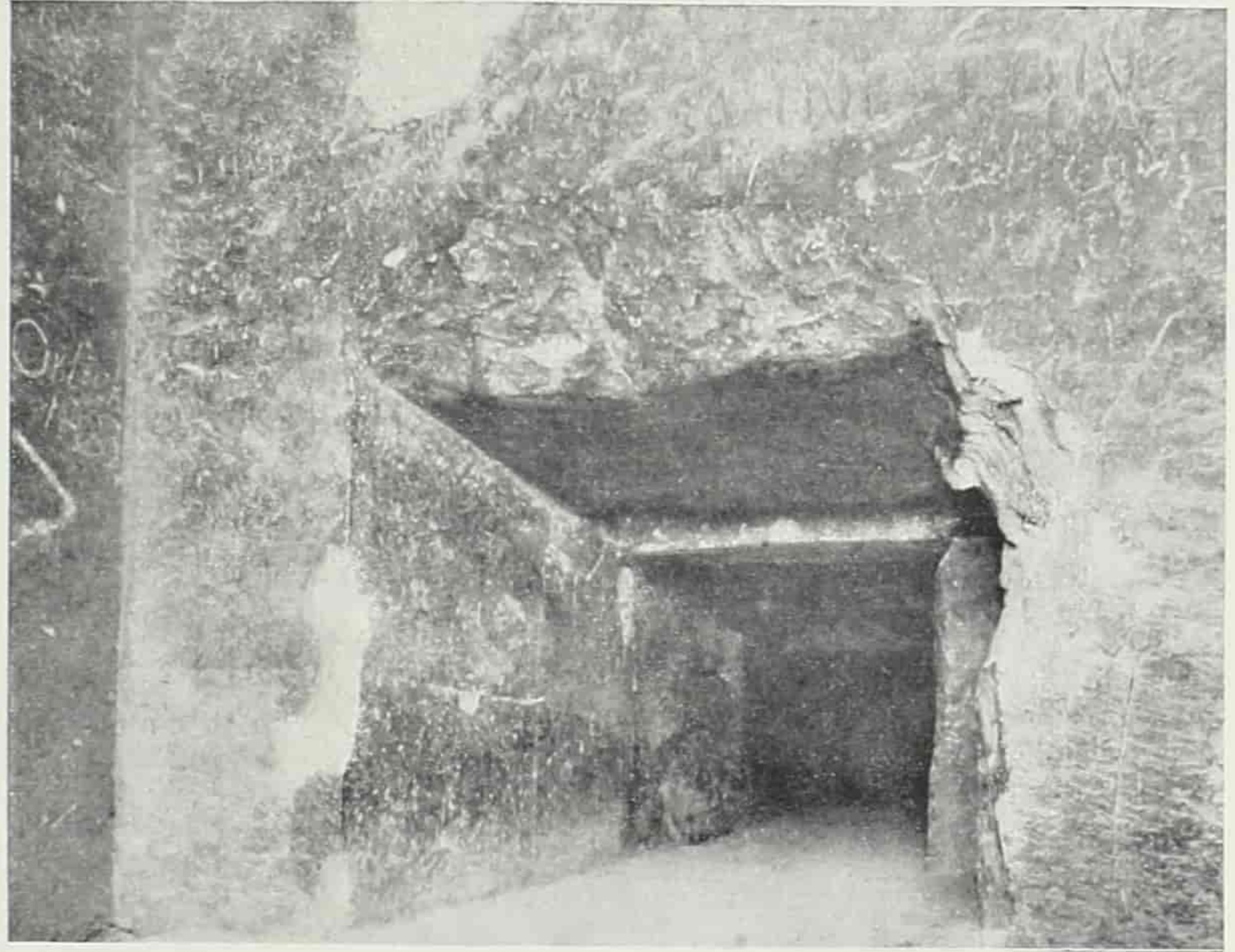
The low passage leading horizontally southward from the Grand Gallery to the Ante-Chamber and King's Chamber.
