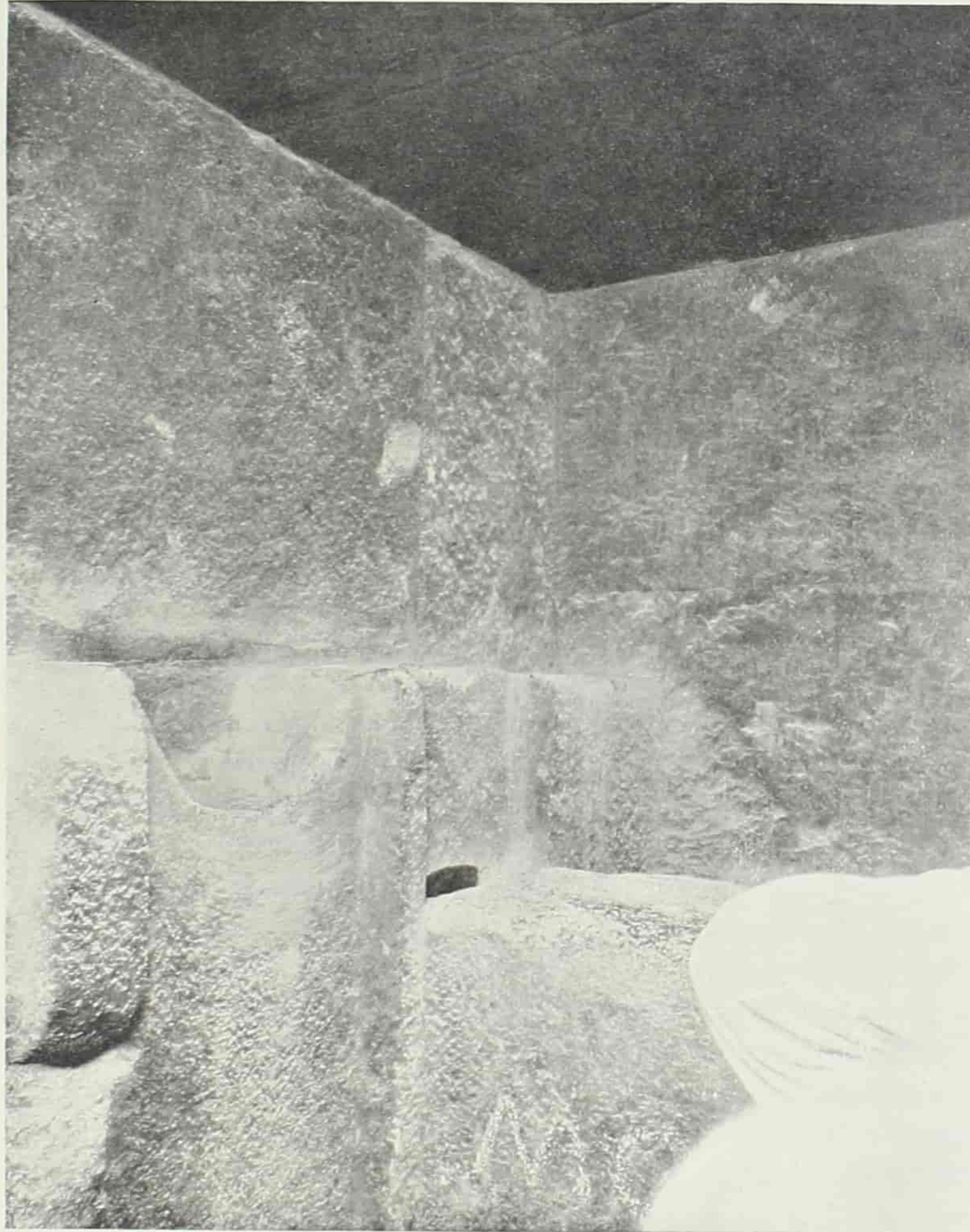
The upper end of the Granite Leaf in the Ante-Chamber of the Great Pyramid of Gizeh; showing one of the three semi-cylindrical grooves in the top of the west wainscot.
