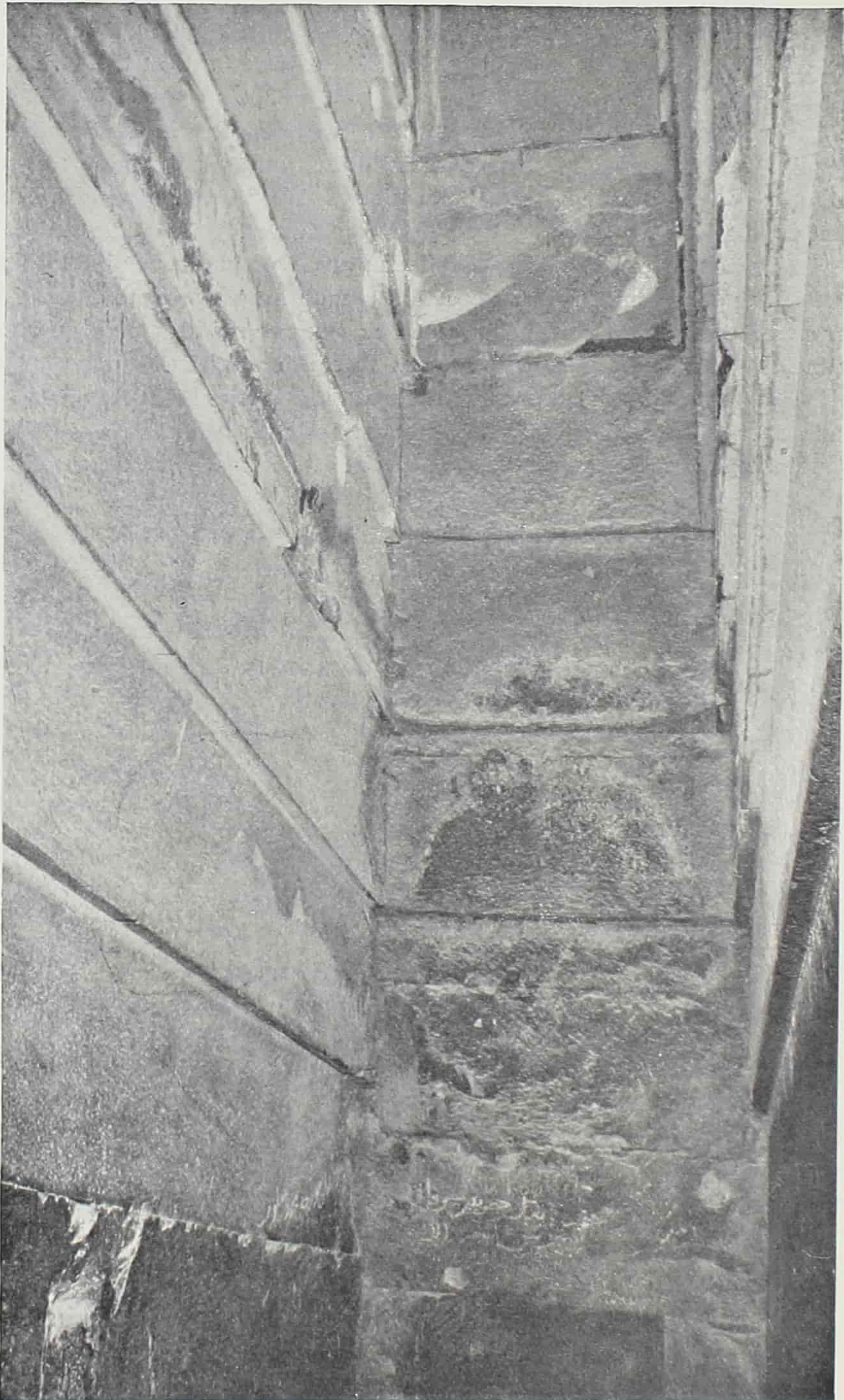
A section of the north end of the GRAND GALLERY of the Great Pyramid of Gizeh; showing six of the seven overlappings of the side walls; also, at the base of the north wall, the upper half of the doorway of the First Ascending Passage.
